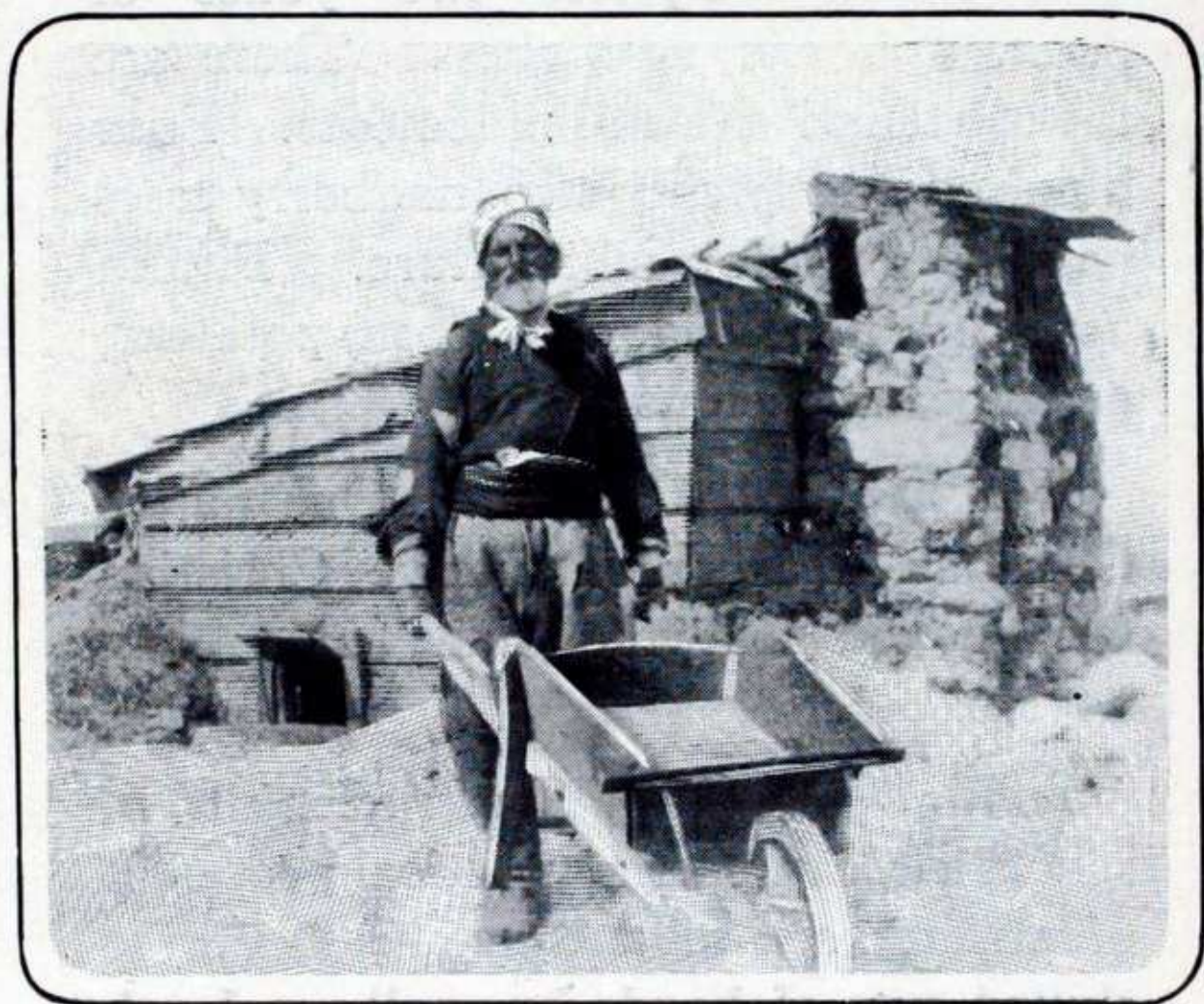
FORMER SHANTY OF CARETAKER
