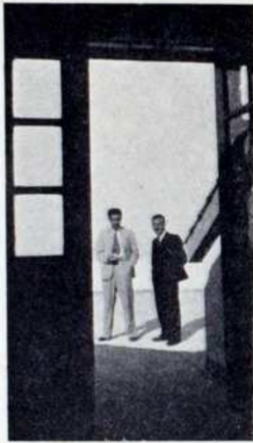
The Terrace Roof.
