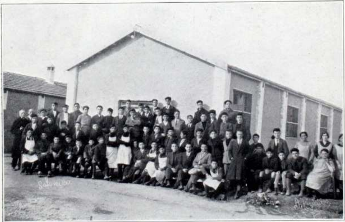
OUTSIDE THE DINING ROOM—BUILDING CONSTRUCTED AS FRENCH MILITARY HOSPITAL WARD
